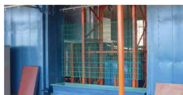
Powder Dip Coating Line China
